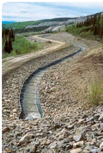
2. Vangorda Creek Diversion.
