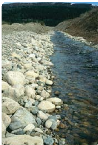
1. Faro Creek Diversion.
